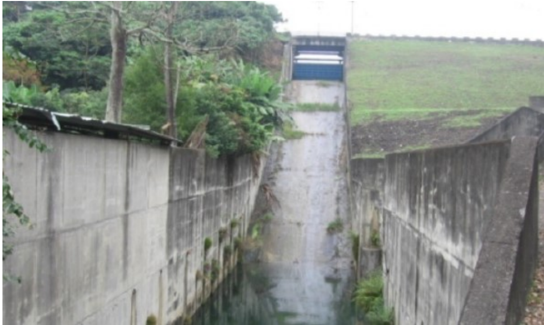
Figure 3. Onsite image of Renyitan Reservoir spillway
