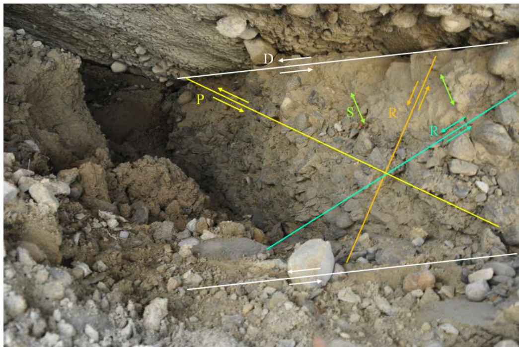
Figure 17. Shear textures existing in the soil beneath sidewall foundations
