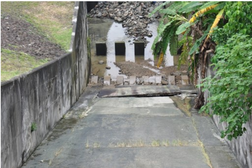
Figure 11. Particles flowing out of Renyitan Reservoir spillway
