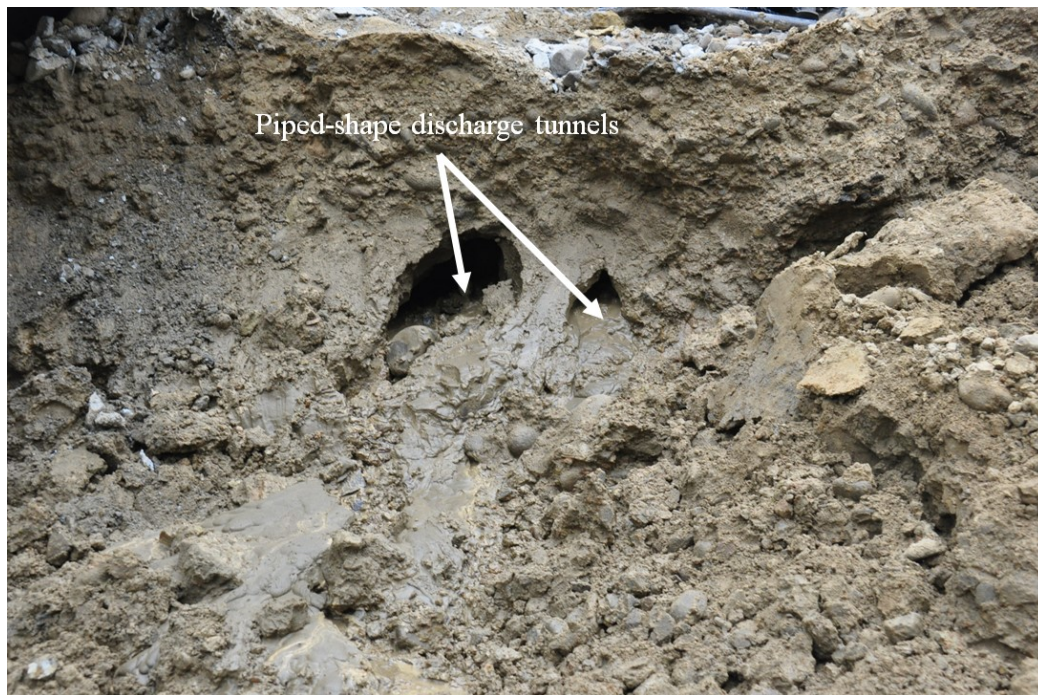
Figure 21. Piped-shape discharge tunnels formed underneath the bottom plate of Renyitan Reservoir spillway
