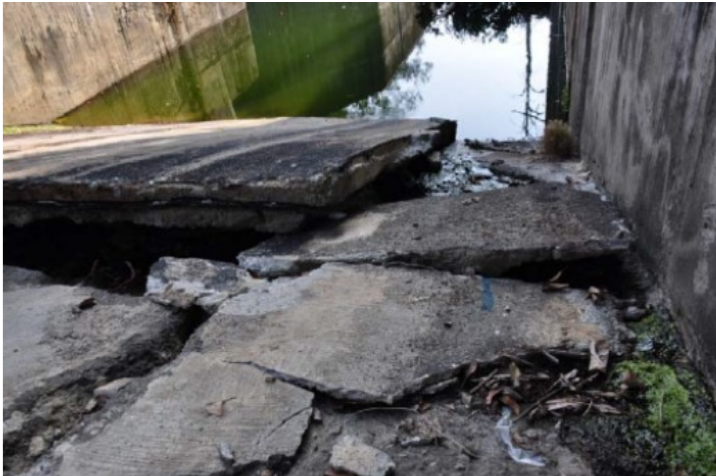
Figure 13. Seepage water flowing out from beneath the sixth bottom plate
