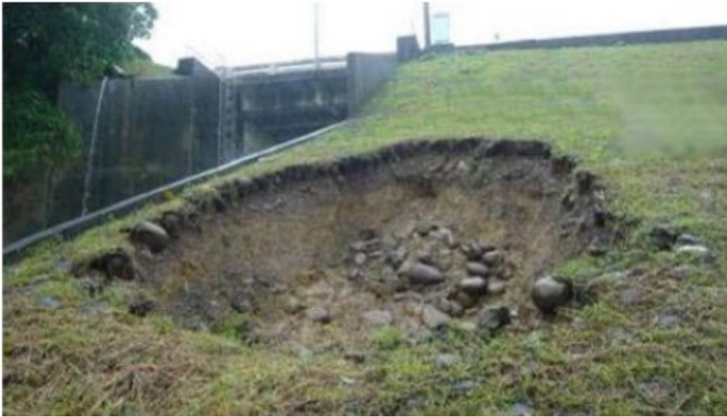
Figure 12. A big piping hole formed at the backside of the wall after piping failure
