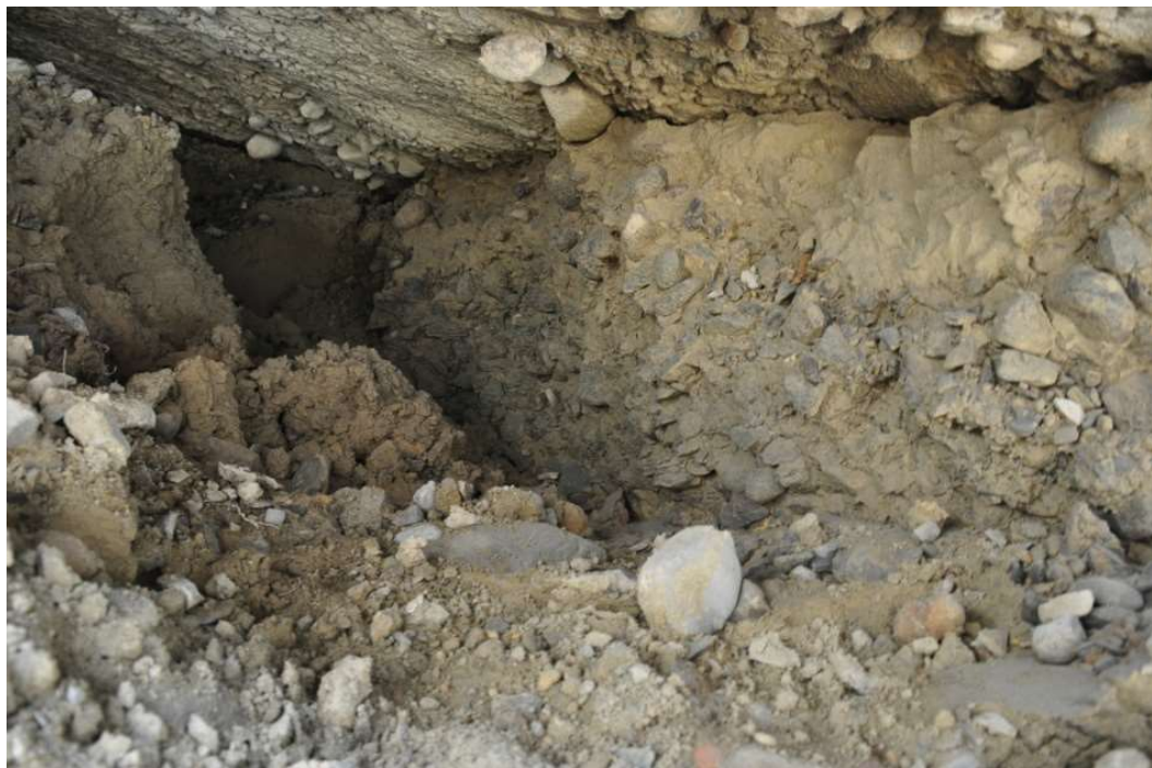
Figure 15. The loss of soil beneath the sidewall foundation of spillway
