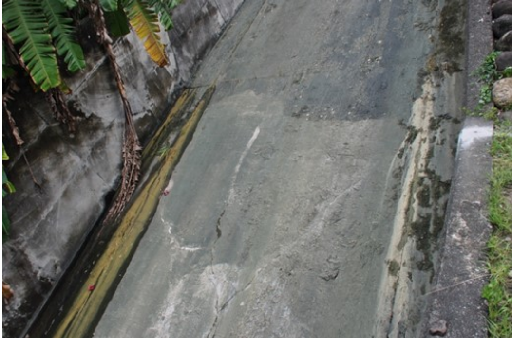
Figure 9. Fracturing of bottom plate and bending of sidewall
