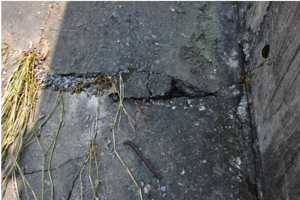
Figure 19. Fracture of sidewall foundation
