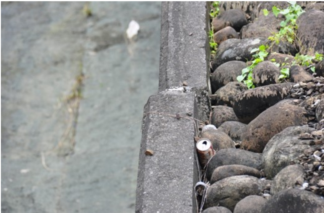
Figure 10. Relative displacement of sidewall
