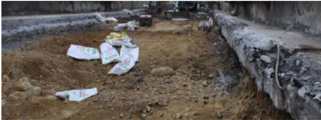
Figure 14. The loss of soil beneath the bottom plate of spillway
